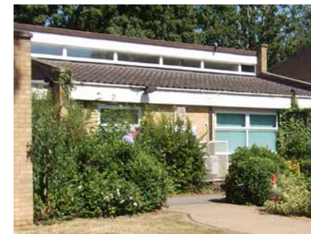
Figure 4.7 Health centre, Exeter Close
