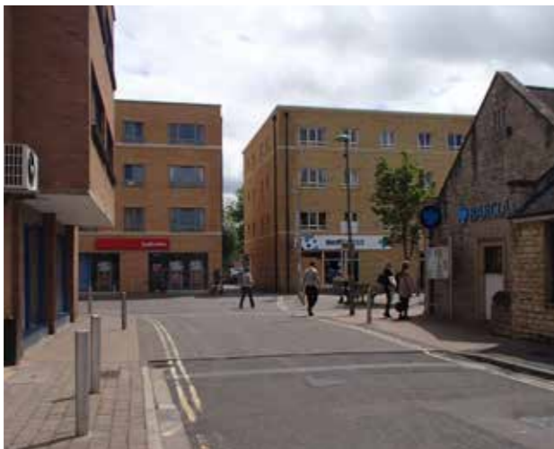
Figure 4.17 Poor quality design of prominent recent schemes
